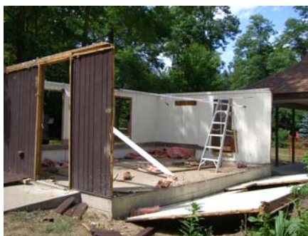
Cabins 2 and 6 were the first cabins to come down.
